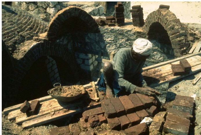
Figure 4. Using mud brick construction techniques, a mason builds an inclined barrel vault (AKTC)
